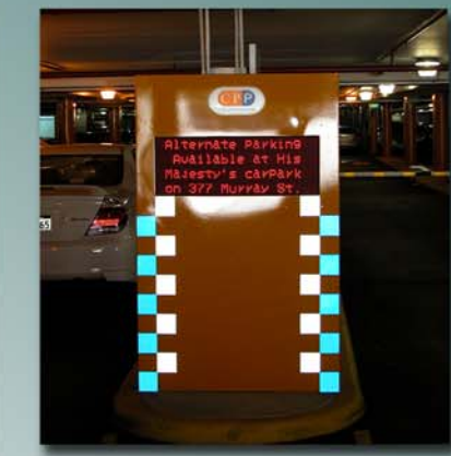
15. City of Perth Car Park Entrance Display
